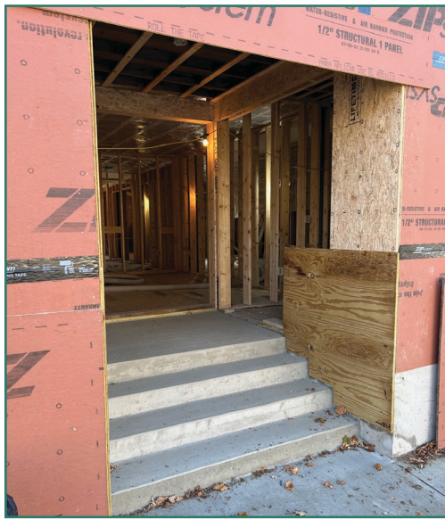
New front entrance stairs, sidewalk and foundations poured.
